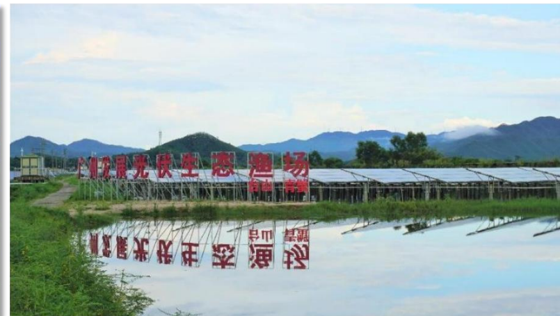
Taishan Photovoltaic Tourist Town (JiangMen, Guangdong) 台山光伏文旅小镇
