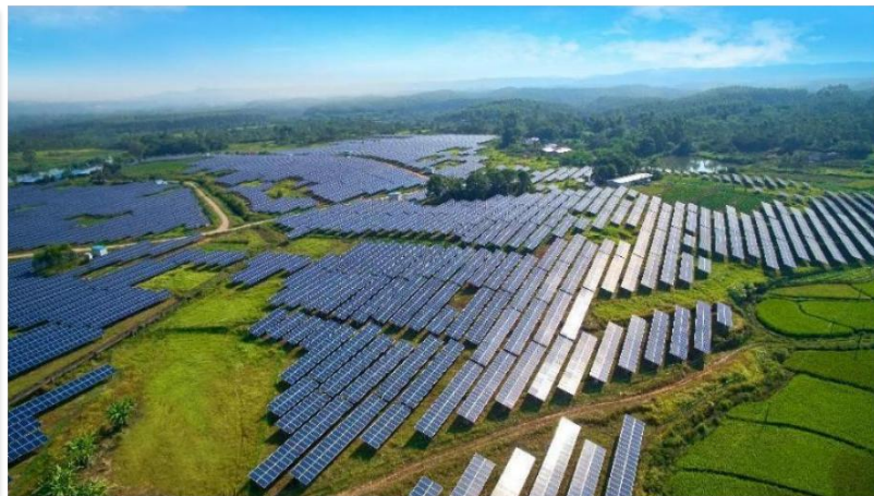
Lianping Agricultural Photovoltaic Project (Heyuan, Guangdong) 连平农业光伏项目
